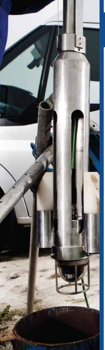
JOHNSONS WELLSCREEN, ZSM STAINLESS STEEL RISING MAIN AND GRUNDFOS SUBMERSIBLE PUMP INSTALLED ON LARGE COMMERCIAL BOREHOLE
